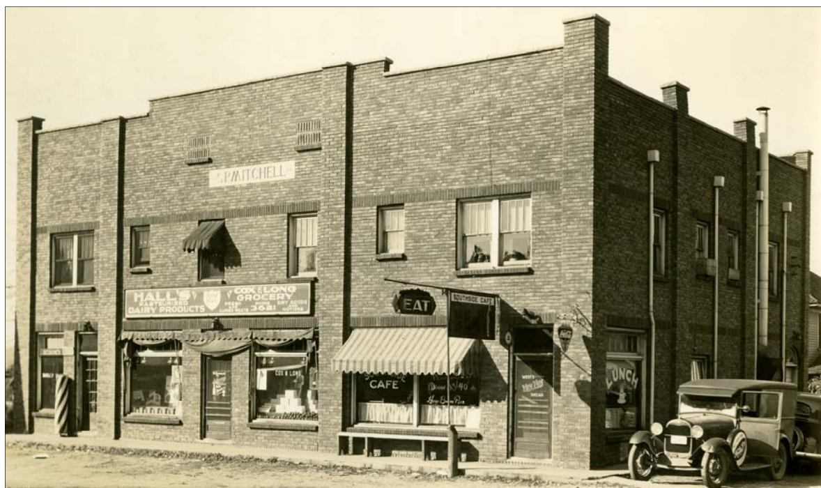
The S. P Mitchell building (built in 1924) housed several businesses, including the South Side Café. From the collection of the Monroe County History Center 1986.077.0207a.
